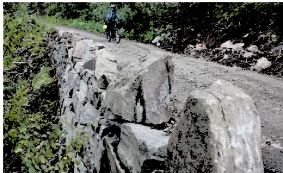
Th: Mur reparert 2015, merk stabbesteinane.
